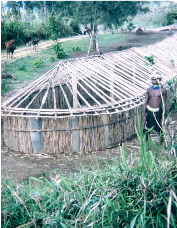
Figure 3.6. Construction of a women's house.
