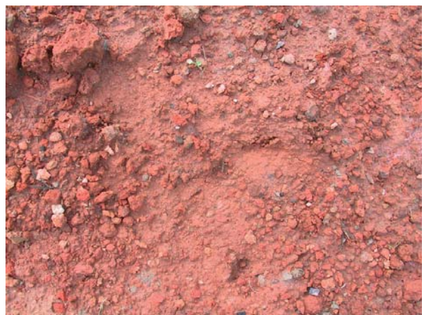
Figure 12.19. The surface of a [collapsed] fired wall.
