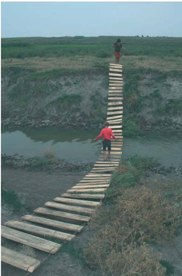
Figure 12.8. The mobile bridge positioned across the Vadastriza river.
