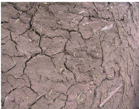
Figure 12.18. The surface of the walls before firing.
