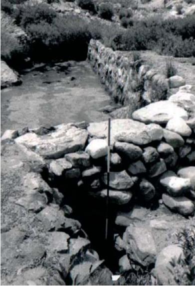
Figure 5.10. Reservoir (tank) and canal outlet.
