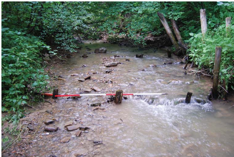
Fig. 6.6. Cigel'ka: wooden constructions in the stream bed.
