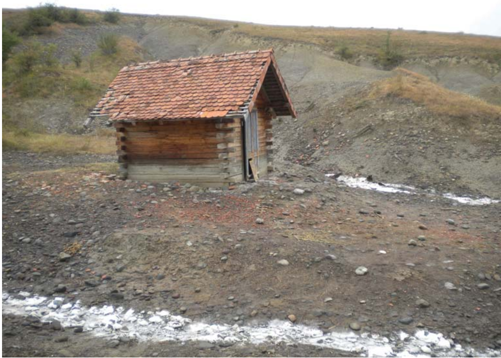
Fig. 4.92. Orşova, brine well house.
